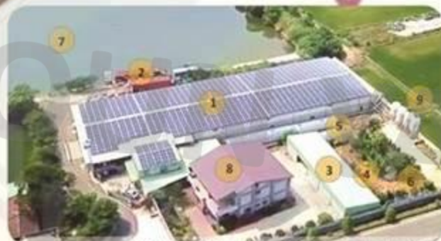
綠能科技 (造肉工廠) Smart green energy technology ( Broiler poultry house / factory )
